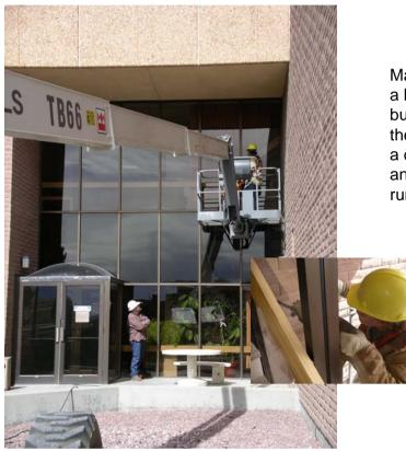
Matt uses a manlift to raise him up so he can drill a hole (inset) through the wall of the control building into the preactivation cabinet that controls the correlator room sprinkler system. He will install a drain to the outside so if there is ever a problem, anyone walking in the front door will see the water running and know something is awry.
