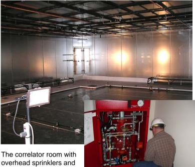
The correlator room with overhead sprinklers and floor racks for the air conditioning system HVAC will install
