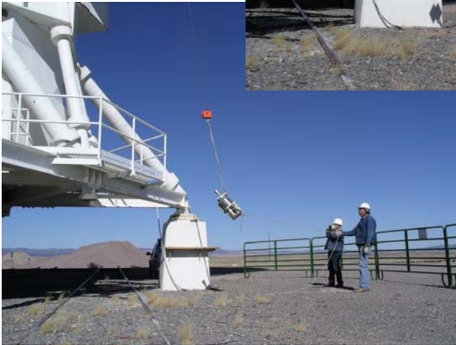
Some of the members of the Front End group are installing a new Q-band receiver in EVLA antenna 13. After they put it in place, the antenna mechanics will realign the feedhorn. It will be turned over to the astronomers to gather data to test it.
